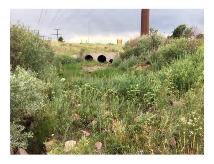
West inlet showing more growth from last inspection. Area was mostly clear from trash and debris. Russian sage should be removed to prevent damning.
