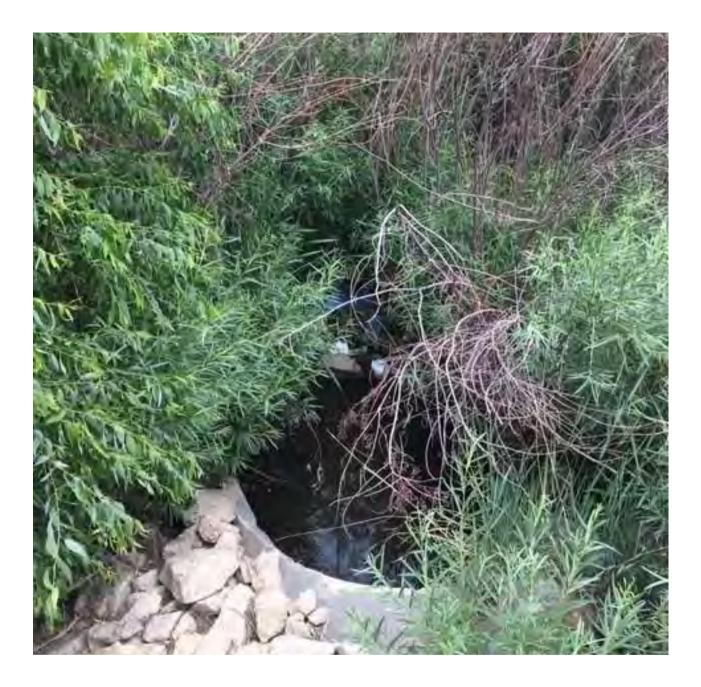
Outlet structure (north-west end of pond). Large amount of sage blocking flow from outlet. This area should be cleared.
