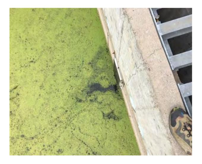
Scrubbed the front plate of the outlet structure to increase flow. More surface vegetation and algae from last inspection has accumulated in the pond.
