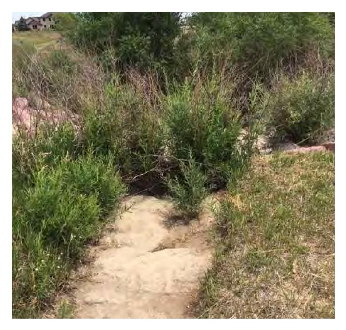
Russian Sage is blocking the inlet to the damn structure/energy dissipator. Sage should be removed to prevent blockage.
