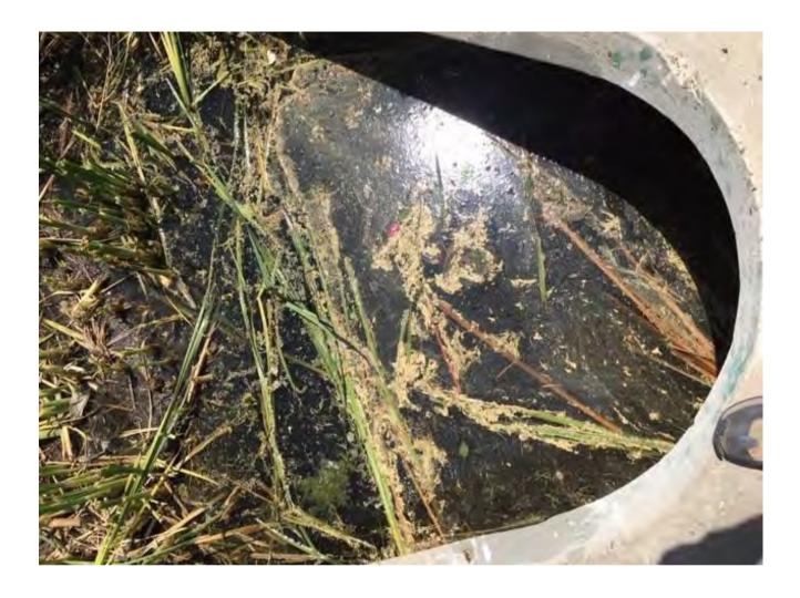
Drainage to Pond J near Mapleton Ct. Large amount of cattails and sage. Cattails in some areas are over 15 feet high. The entire area should have sage and cattails removed. Some damning has already occurred and could lead to flooding.
