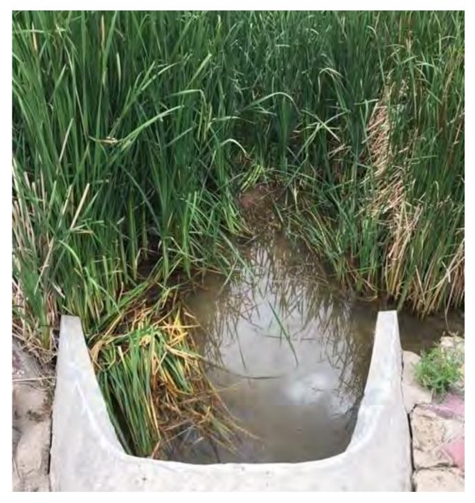
Northern most inlet has significant plant matter and mud at the mouth of the inlet. May need to be removed to prevent future damning. Cattails should also be cut back and removed.
