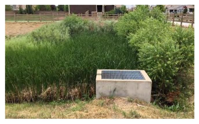
Large amount of cattail and sage growth blocking inlet structure (West end of pond). Area should be cleared. (Below)
