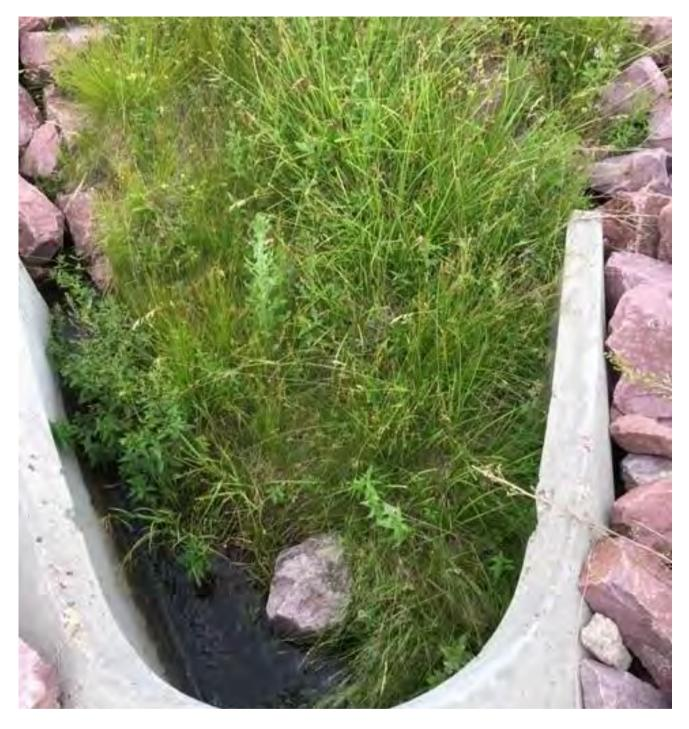
The west inlet has significant growth in and around the mouth of the inlet. This should be removed to prevent blockage.
