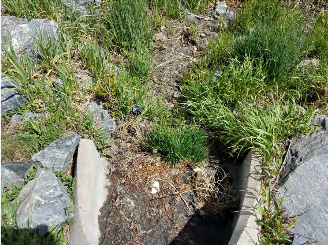
Drainage to J Pond
